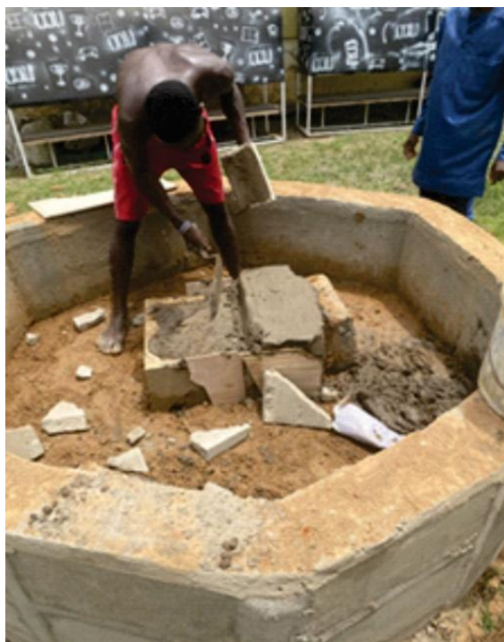
Figure 5. Building the water fountain basin. Medium: Sandcrete blocks, concrete
