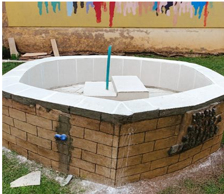
Figure 7. The interior part of the water fountain basin is piped and fully tiled. Medium: Sandcrete blocks. Concrete, ceramic wall and floor tiles. Size: Length (1143 mm), Breadth (203 mm), and Height (686 mm) for each side of the hexagon
